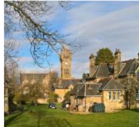
General view towards Mount Zion Church
