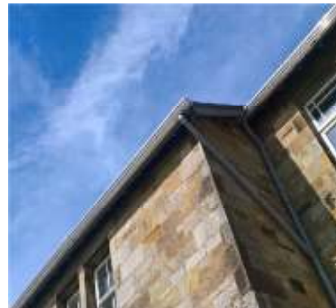
Aluminium guttering in use at the hall
