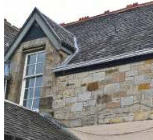
Replacement guttering in aluminium
